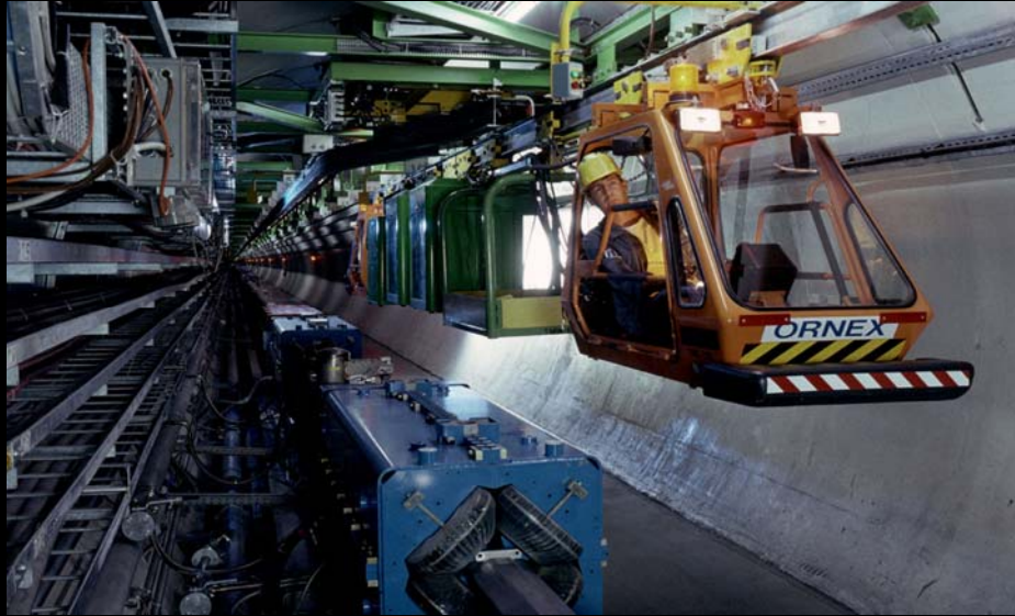
Inside A Circular Particle Accelerator Tunnel : Monorail !
